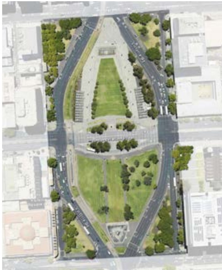
Figure 60a - 2021 Victoria Square aerial photograph. Source: Location SA
